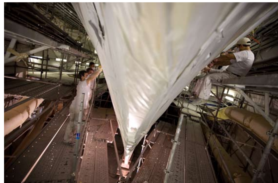
Above: Constructing the interior is a highly complex task.
